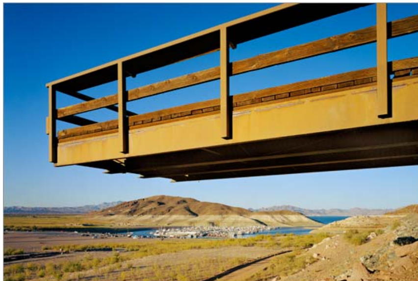
A pier to nowhere at Lake Mead Marina. Water Levels are near historic lows and getting lower.
